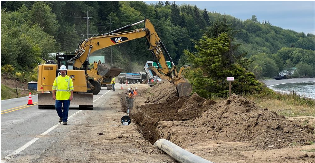
District water crew works on BU 945 Clallam Bay-Sekiu Infrastructure Upgrade.
