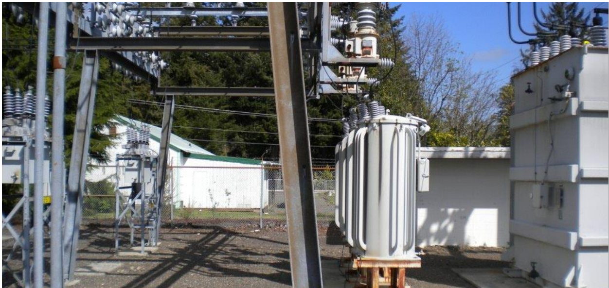
BU 207 Forks Rebuild & Reconsolidation
