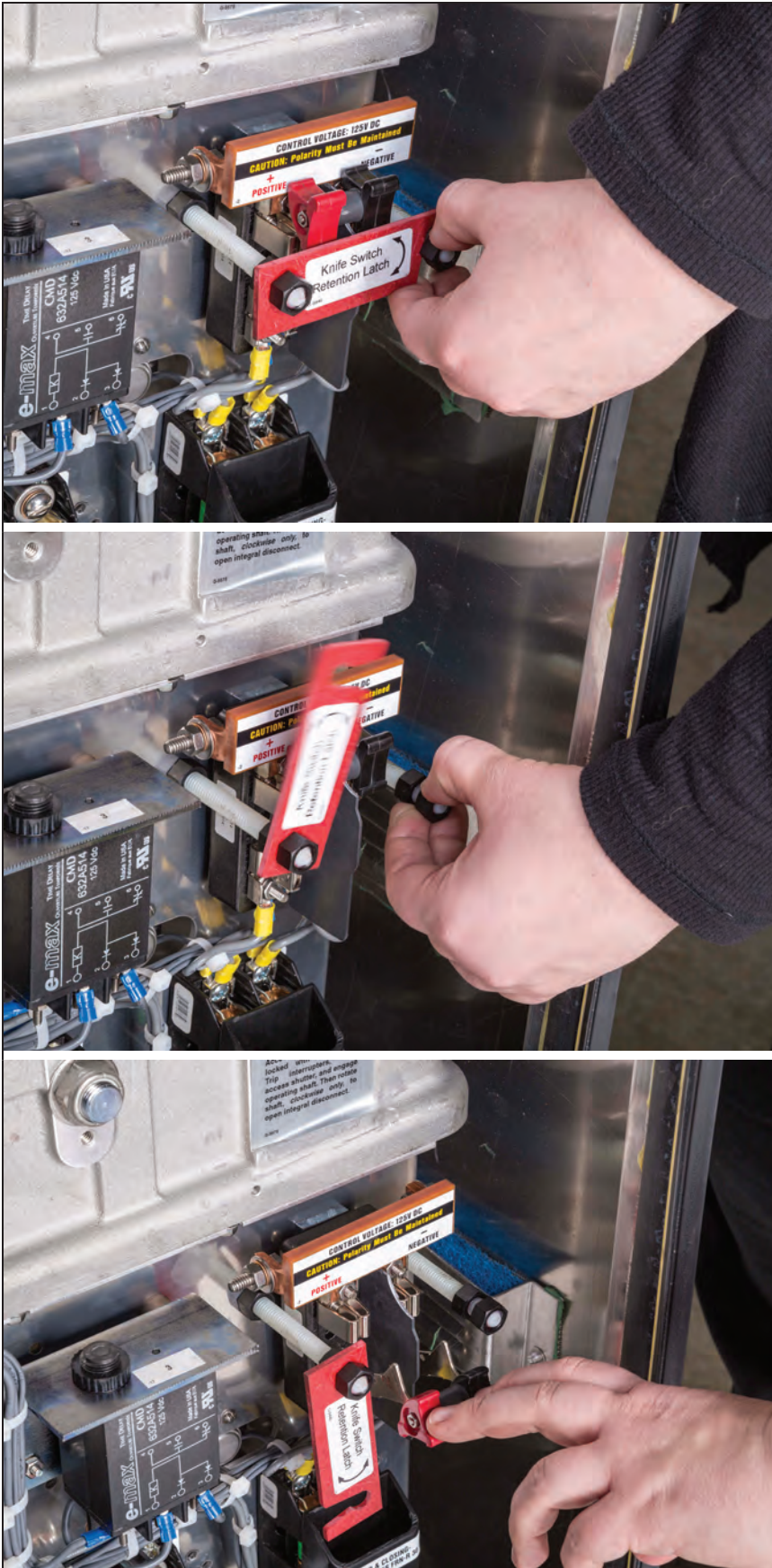
Figure 25. The knife switch retainer and knife switch.
