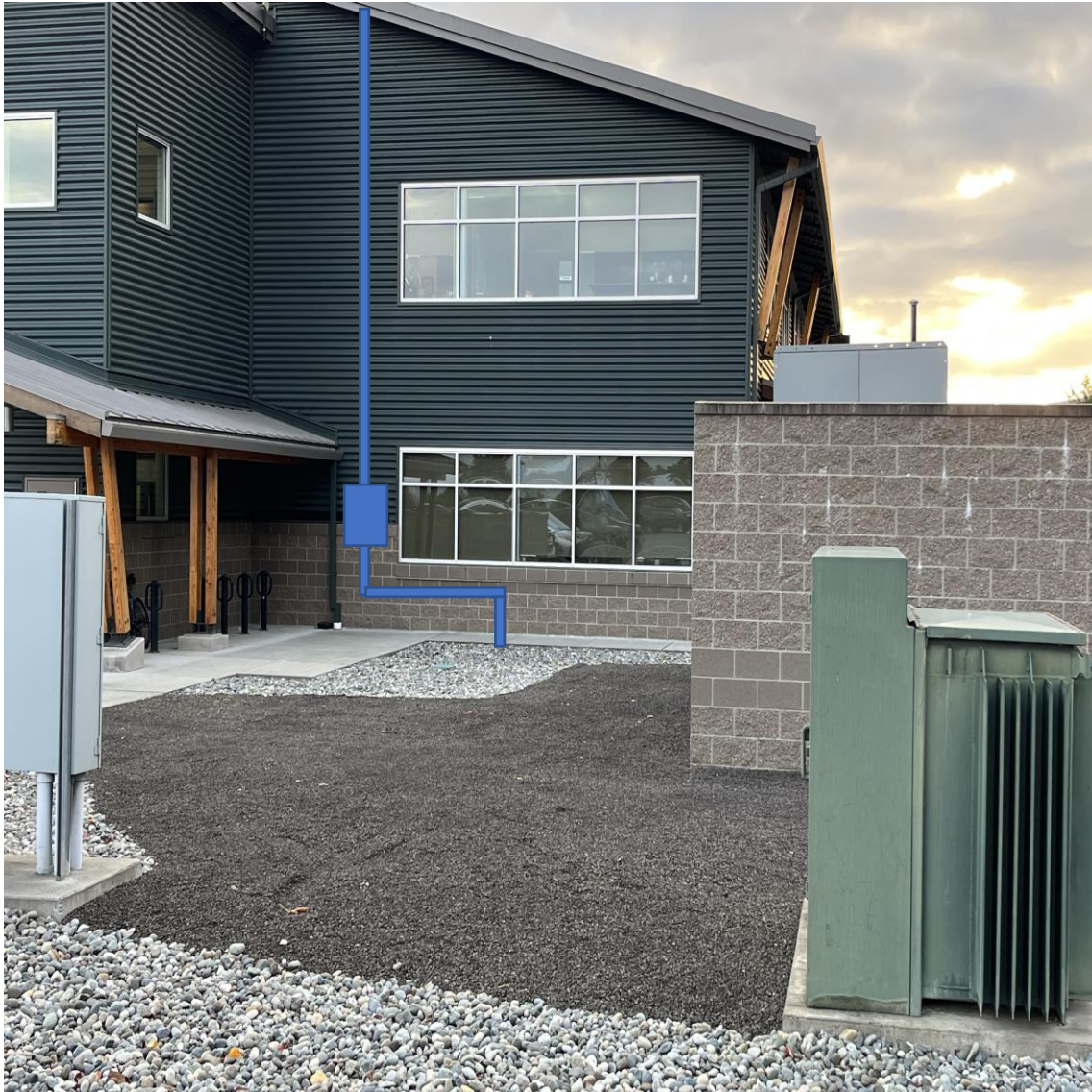
Conduit and Inverter suggested route
