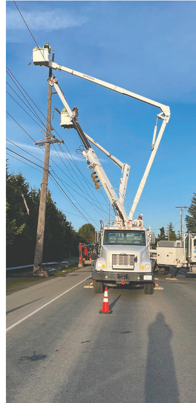
Crews repair damage caused by a car vs. pole accident.
