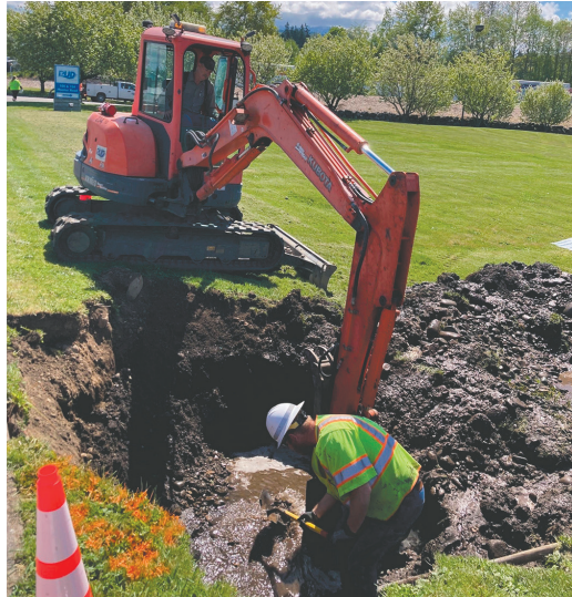
A water main break in Carlsborg required skilled excavating to locate and isolate the break.
