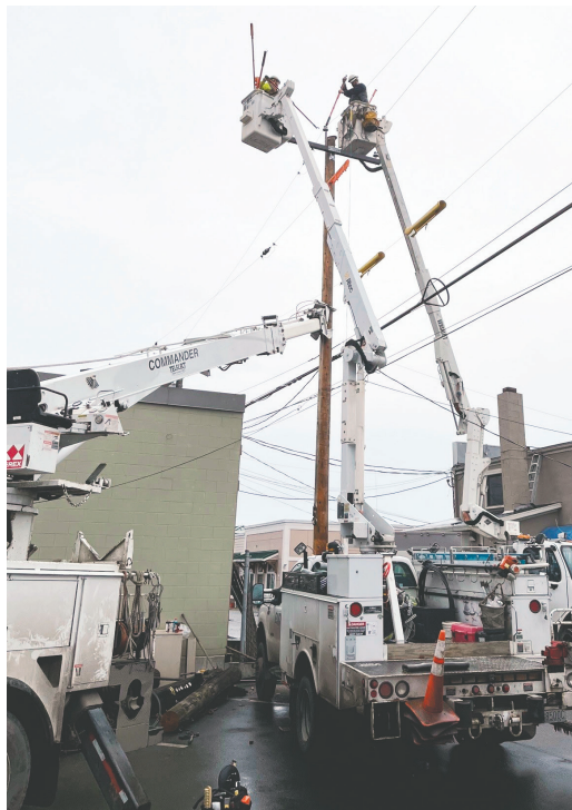
Crews work to replace a broken pole caused by a car vs. pole hit-and-run.
