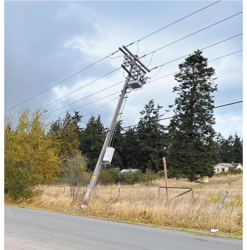
Storm-damaged poles on Gilbert Road.
