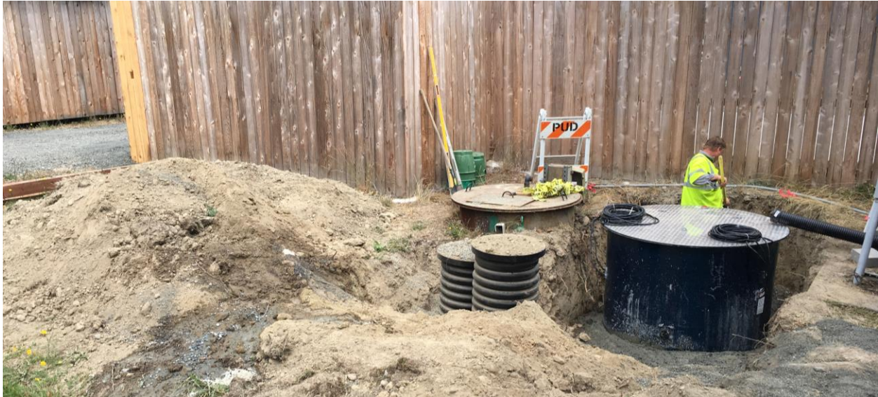
Example of work performed at the upper lift station replacement
