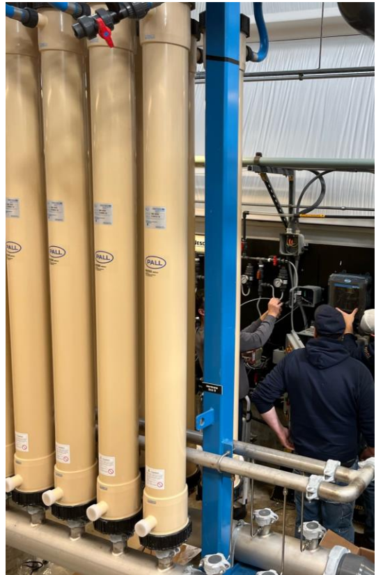
Example of work completed under BU 909.24
