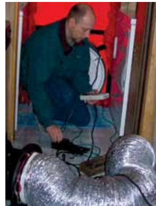
Duct Blaster® testing for leaks.
