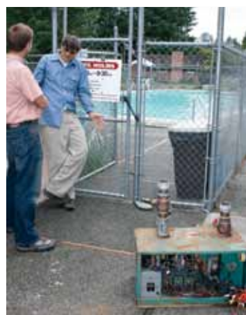
Completed: Custom Commercial Energy Efficiency Program Project
